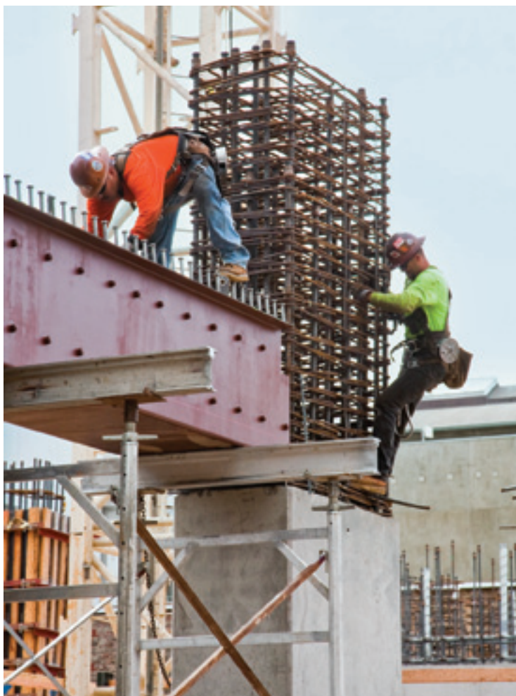
NOVEL LINK Steel-and-concrete link beam needs no diagonal rebar.
