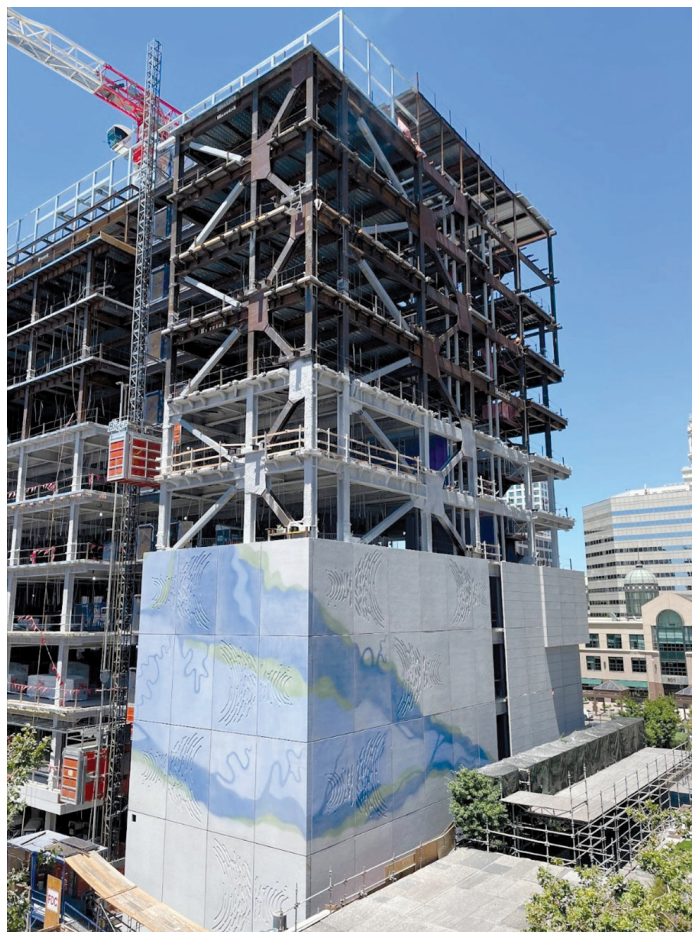
Mast frame construction with facade and fire proofing partially installed.
