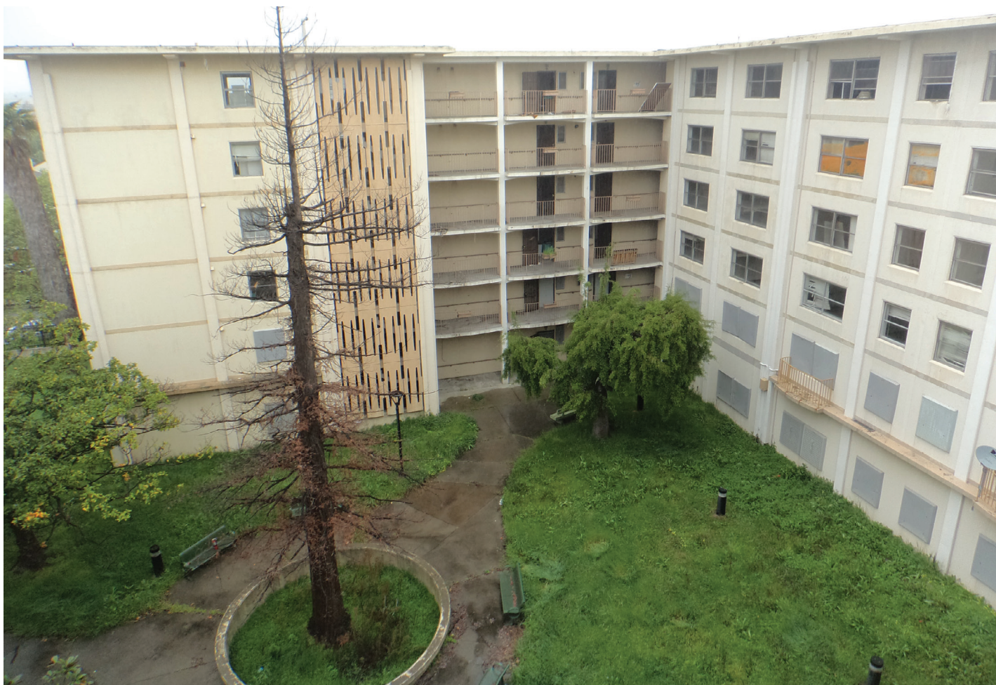
The Hacienda Apartments is a 150-unit complex built in 1964, before modern seismic building codes were developed. (Photo Credit Pyatok)
